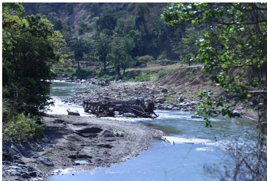
Remains of a bridge over Jupilingo River in Guatemala, destroyed by Eta and Iota in 2020. Photo: José Carlos Rivera.
