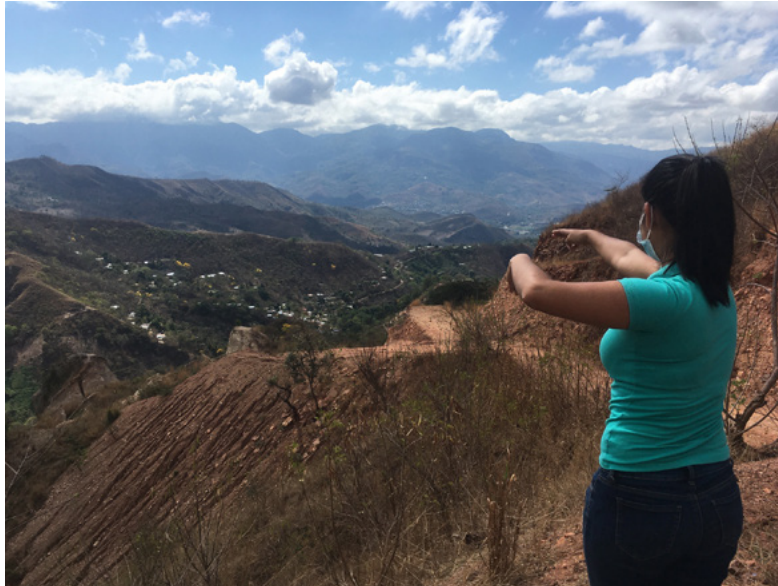
CRural roads damaged by storms in Chiquimula, Guatemala. Photo: Larissa Soto.
