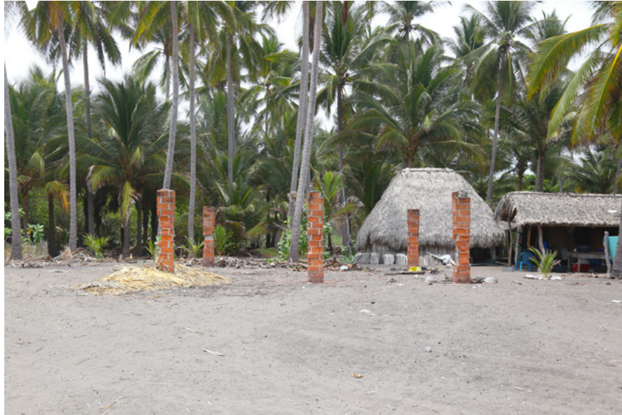
Remains of a house destroyed by a storm surge along the Salvadoran coast. Photo: José Carlos Rivera.
