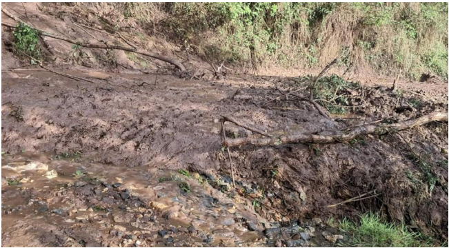
Photograph 6. From the P51 database. Landslide in Guatemala
